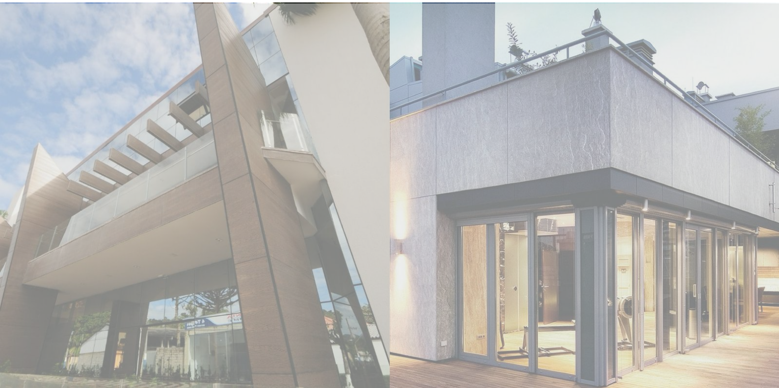
Fiber-cement boards, part of Eternit's Industrialized Construction line, used in façades of commercial and residential buildings
