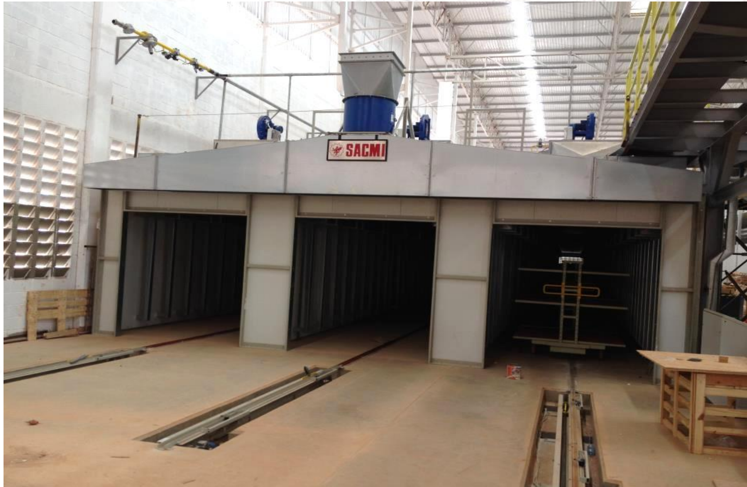
Finalization of the drying
