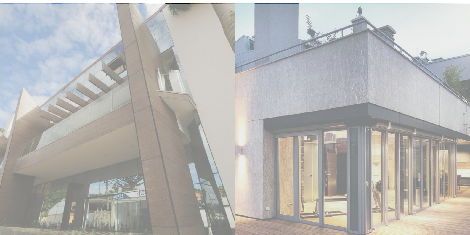
Image 10: Cement Cladding Panels, products that make up the Eternit Construction Systems line, applied to the facades of commercial and residential buildings.
